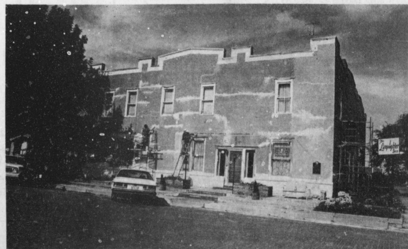
RESTORING HISTORY--David James and his painting crew have been hard at work restoring The Lamplighter Bed and Breakfast to its original grey color with white trim. The windows will feature black trimmed screens. Roxanne Cummings and Evelyn Branch, owners of the
