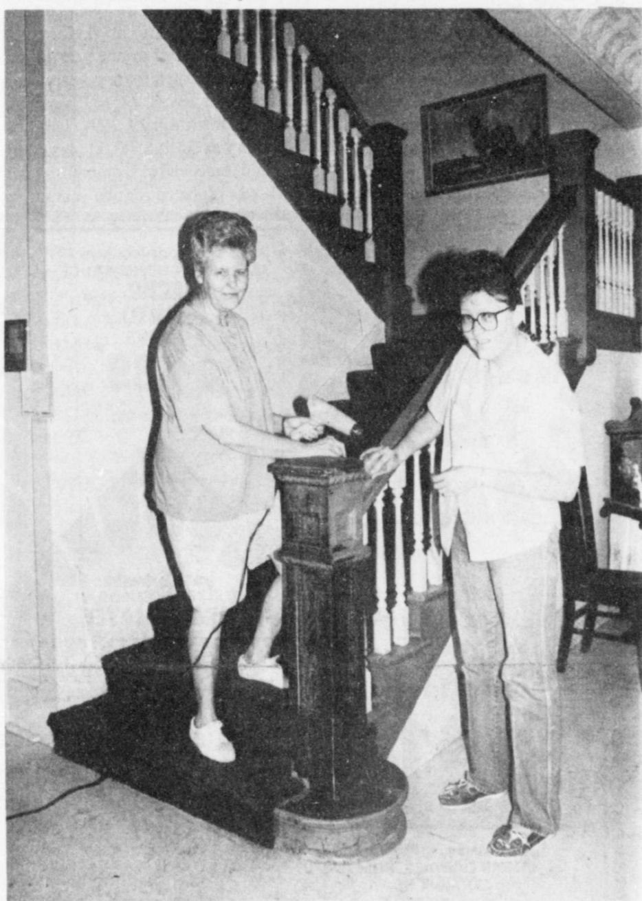
LAMPLIGHTER RENOVATION UNDERWAY--Evelyn Branch (left) and Roxanna Cummings, new owners of the Lamplighter Inn, are hard at work renovating the historic structure in preparation for opening it as a bed and breakfast establishment. --Staff photo
