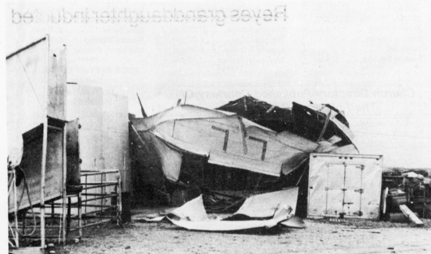
WHAT A MESS -- Damage from last week's storms included the quonset barn at Sam Fortenberry's place south of Lockney. Pulled apart by high winds of possible tornadic nature, pieces of the barn damaged the roof of the family residence. The wind driven rubble stacked up against these tanks when it final came to rest. Staff Photo
