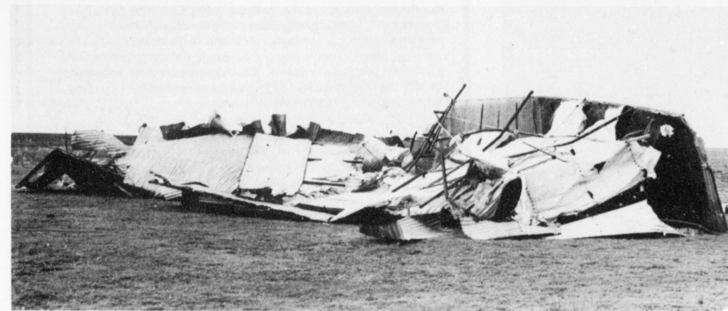
FARROWING BARN LOST --This farrowing barn at Ellis Butler's home, east of Lockney, was ripped from its foundation and left in a crumpled heap two hundred yards northeast of its original spot. The barn was anchored
