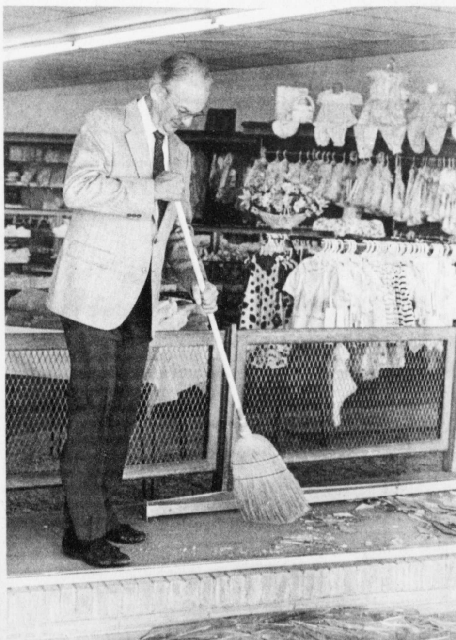
DRIVE THRU DEPARTMENT STORE --Claude Brown, owner of Brown's Department Store in Lockney, stands on his front display platform and sweeps glass from his storefront window after a Lincoln Town Car, driven by a Lockney woman, drove through the front windows. The driver of the vehicle accelerated into the window after her car was struck from behind, on Monday, April 29, at approximately 9:30 a.m. No one was injured in the accident. The vehicles sustained minor damage.
