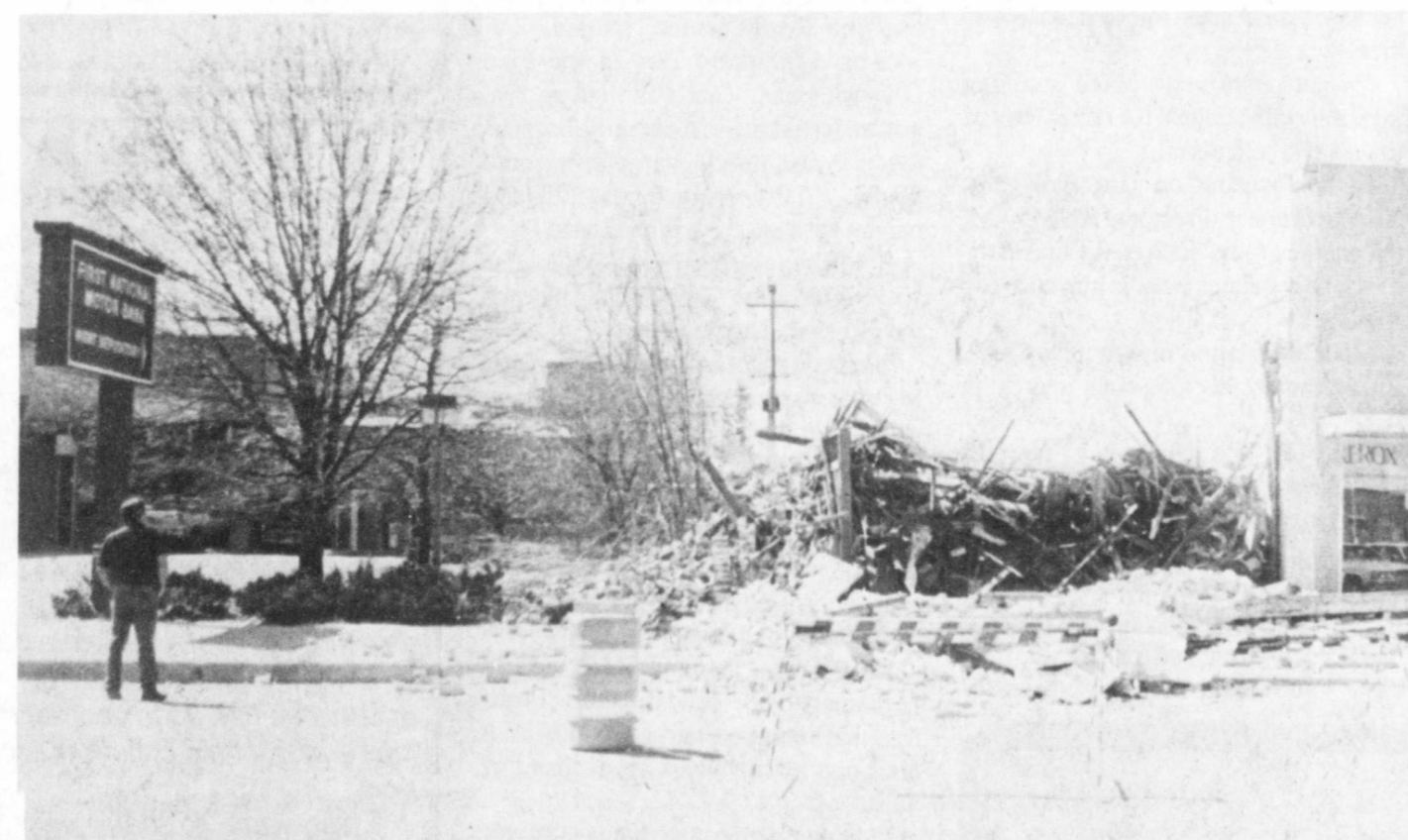
LANDMARK IS GONE—Keith Marricle (at left) looks at what's left of a landmark that was torn down Saturday and Sunday, March 17 and 18, because of the fear it might fall down someday. The building was owned by Ronnie Wayne Day, and located on the south side of Script Printing, 110 S. Main. The building has housed the H.J. Willis Hardware and Furniture Store in the 20's; a cafe (on the bottom floor) and a hotel on the top floor in the 40's. A
