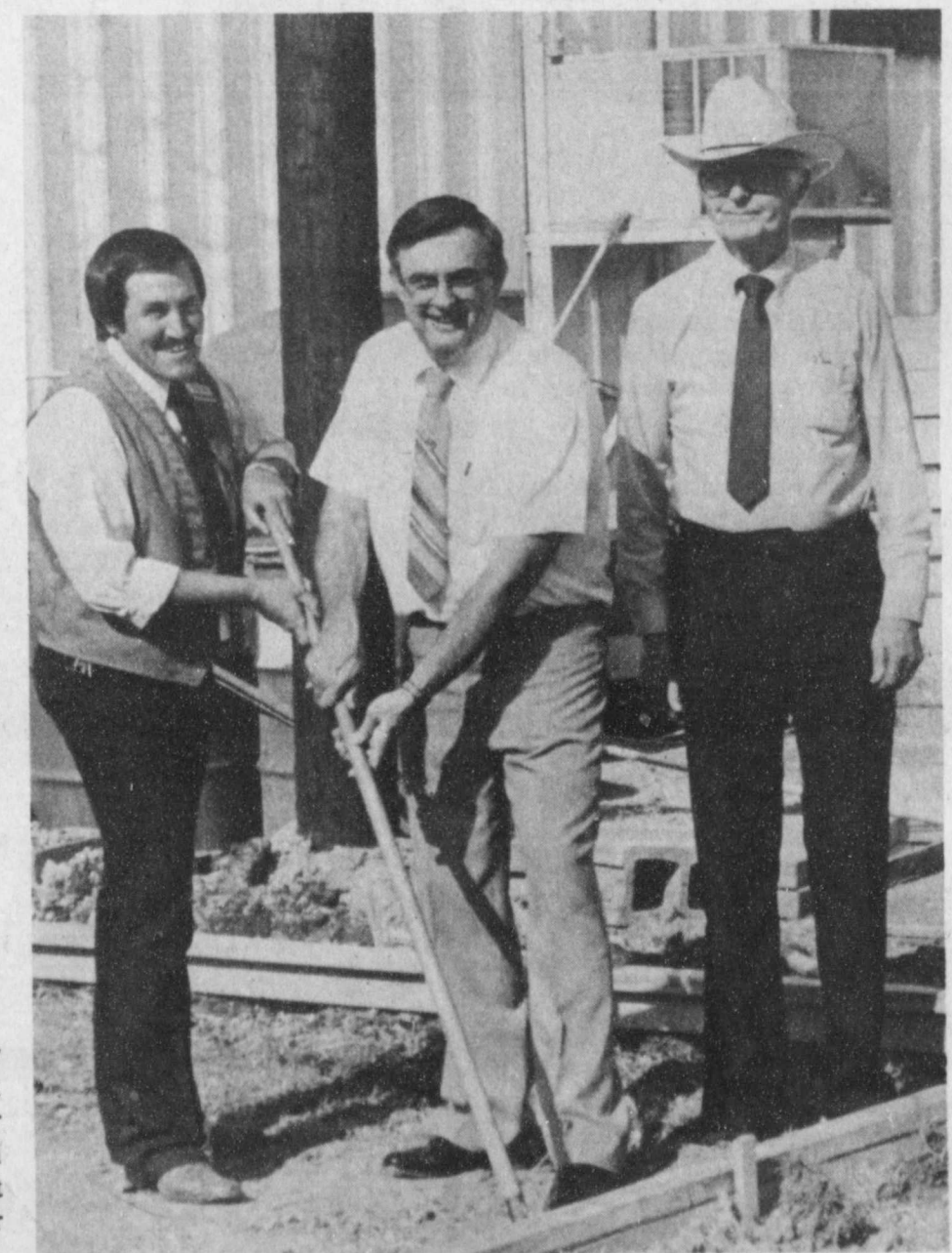
BREAKING SOIL —(left-right) Local Pay-N-Save manager Johnny Summers and owner Roger Lowe are joined by Mayor Parnell Powell, in breaking new ground in preparation for expansion at Pay-N-Save. "The construction should be completed by November," said Summers. "We will have a bigger parking lot and with the extra room we will be able to carry a larger variety of merchandise. We will have a larger produce, frozen food and meat department. With all the new merchandise and the wider aisles we feel we will make the store more convenient for shoppers." Staff Photo
