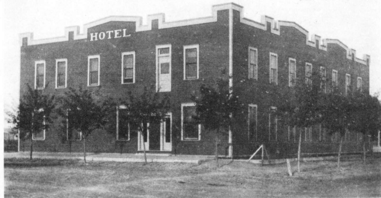
COMMERCIAL HOTEL — This picture, taken in the early teens, depicts the beginning of the guest house later to be named the Lamplighter Inn. A ceremony to dedicate a
