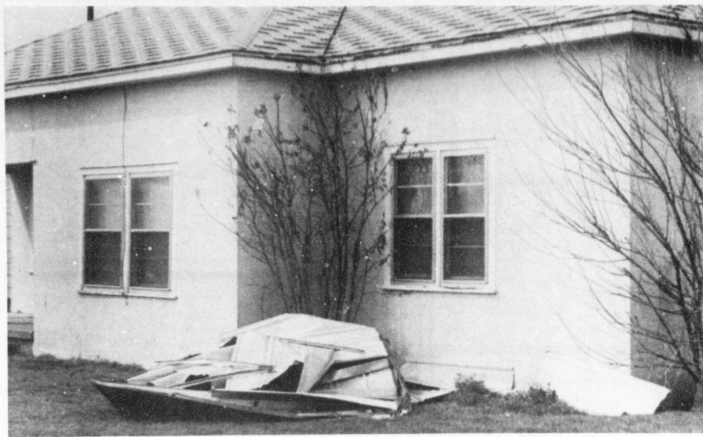
FORMER SHED?—What appeared to be pieces from a small shed, apparently devastated by Monday morning winds, were scattered against a residence at 322 West Missouri. —Staff photo
