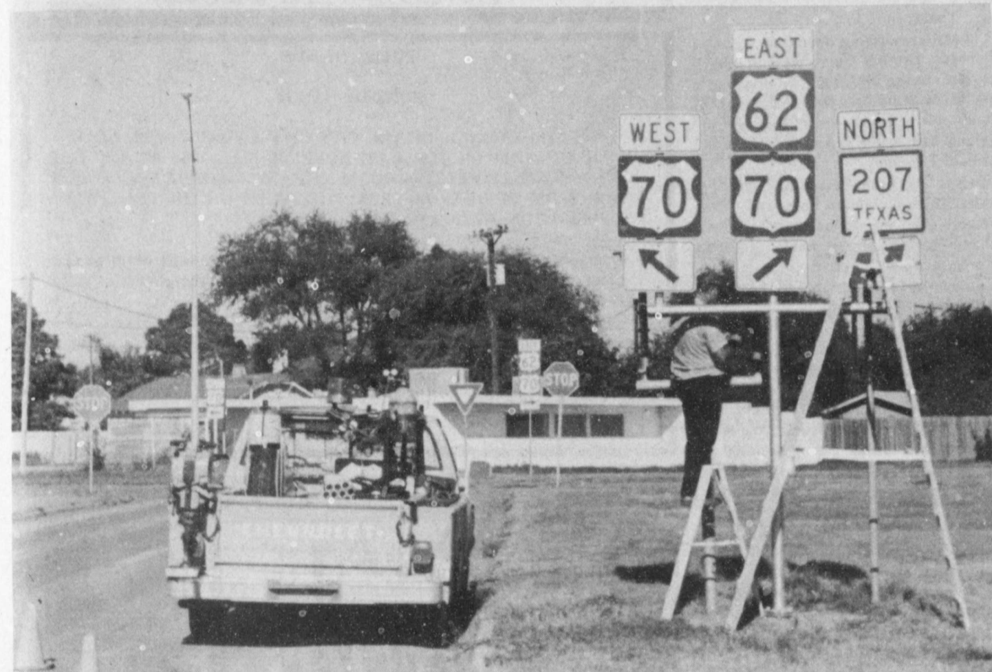
CROSSROADS — Gordon Hambricht of the State Department of Highways of Public Transportation converts the double to single post style for signs in the southwestern part
