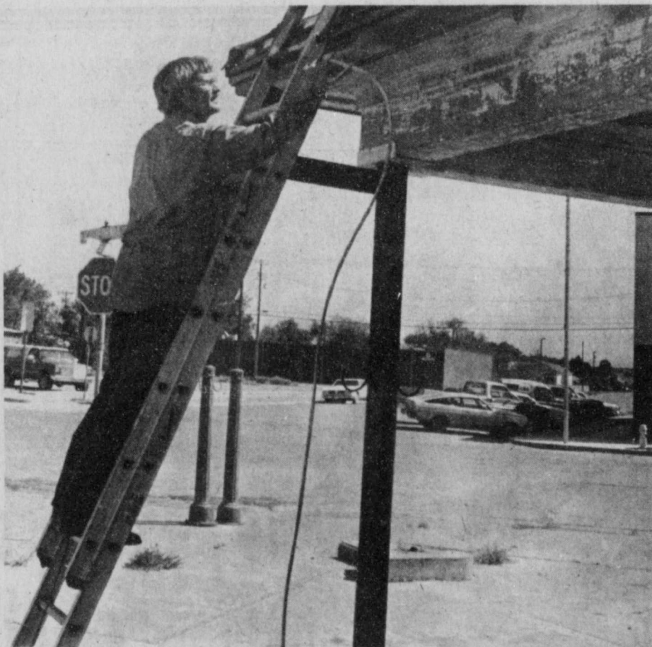
COVERALL CORNERS is the new business moved into 202 W. California. Mr. A.T. Thrasher and his wife, Candy have already opened their combination upholstery, gifts and antique store. Mr. Thrasher is giving the old building a new look that has already brightened up that once deserted corner. The grand opening of Coverall Corners is planned for Memorial Day.
