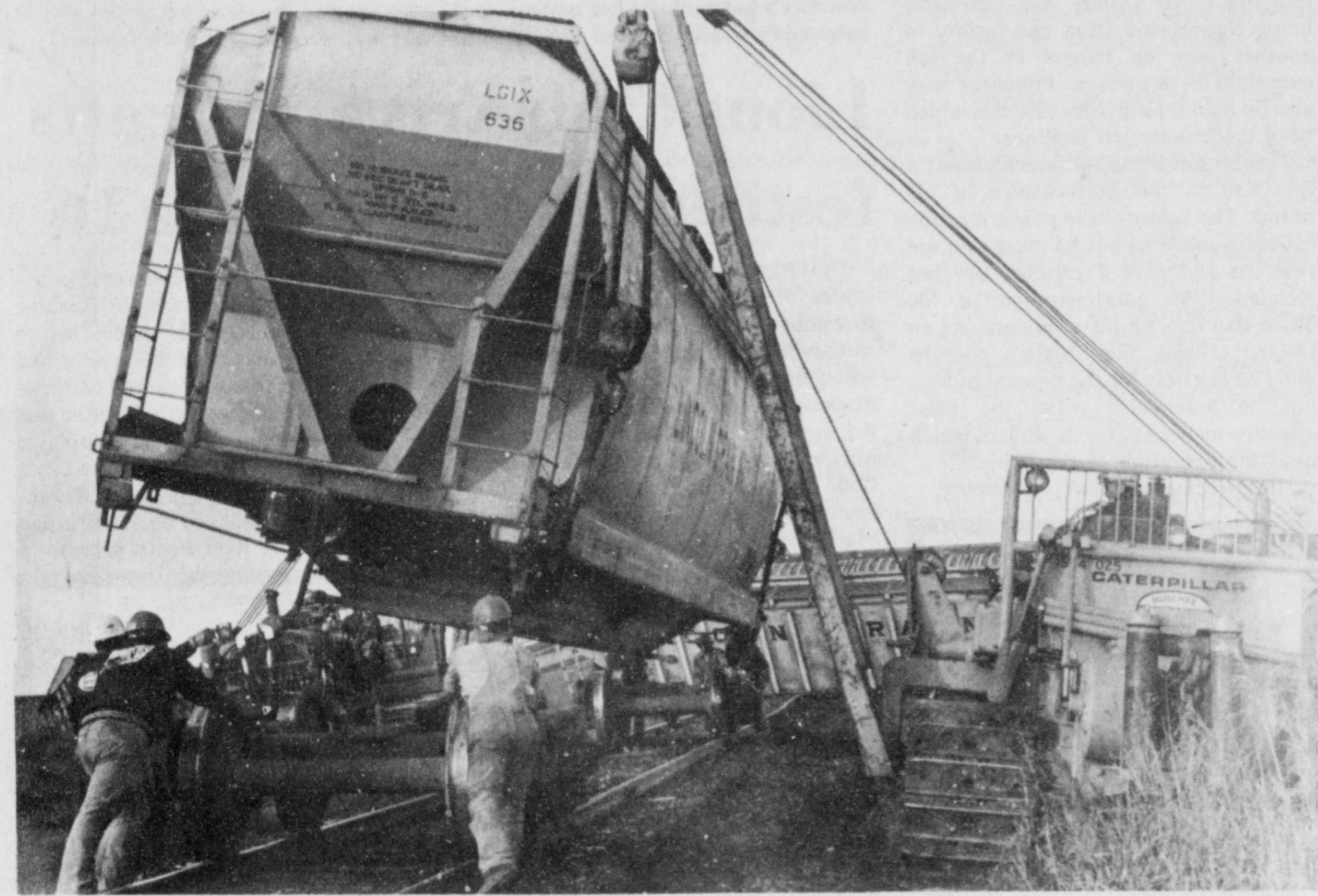
BACK ON TRACK —Hulcher Emergency Services of Amarillo used a variety of special equipment, including 2 cranes, to get 9 empty grain cars upright and back on the tracks after their derailment near South Plains. The clean-up operation took most of the day last Saturday.
