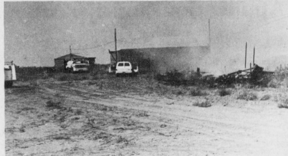
SHED DESTROYED —The smoking remains of a shed destroyed by fire on August 29 are evident in the foreground. The second fire was behind the barn in the center of the picture.
