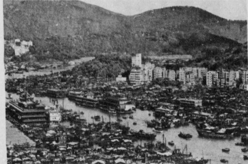
SOME 5,000 "BOAT PEOPLE" live at Aberdeen Bay, down from several million. The government is relocating the families into Federal Housing apartments. Many of their ancestors lived and died without ever having touched their feet on soil.
