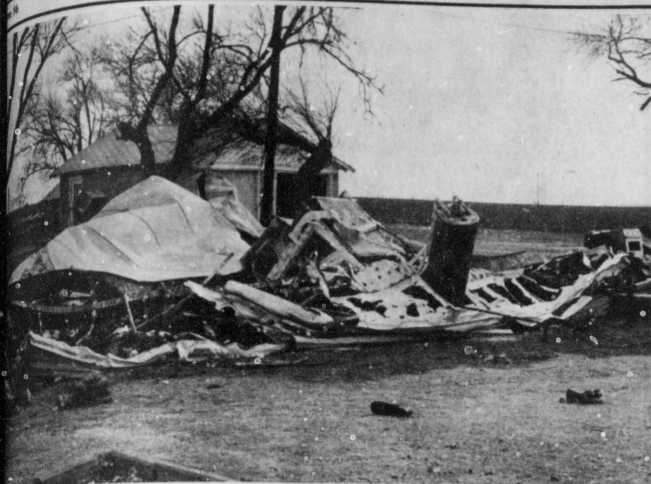
DESTROYED THE LLOYD POOLE mobile home, outside of the McCoy Community. Center photo shows a refrigerator reduced to half its size by the intense heat of the fire.
