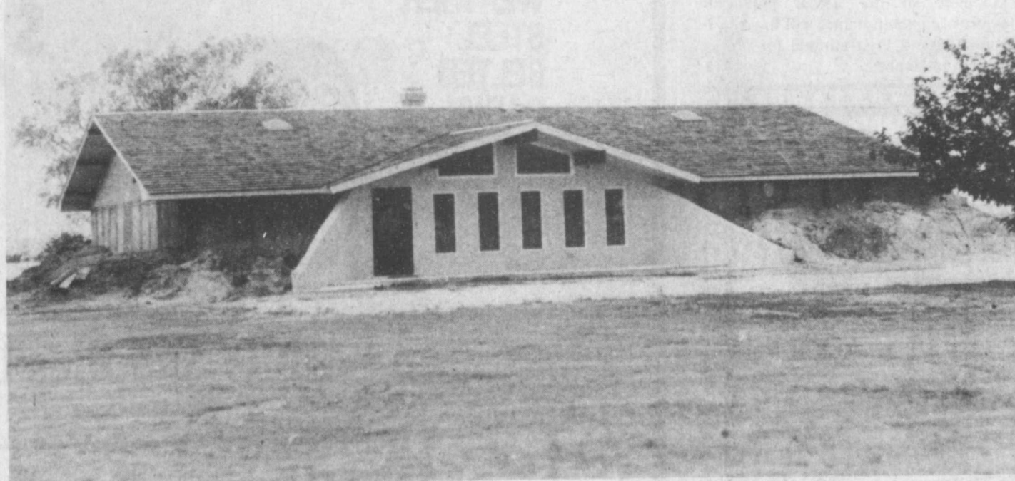
THE EARTH-SHELTER home of Mr. and Mrs. D.L. Miller as seen from the front.
