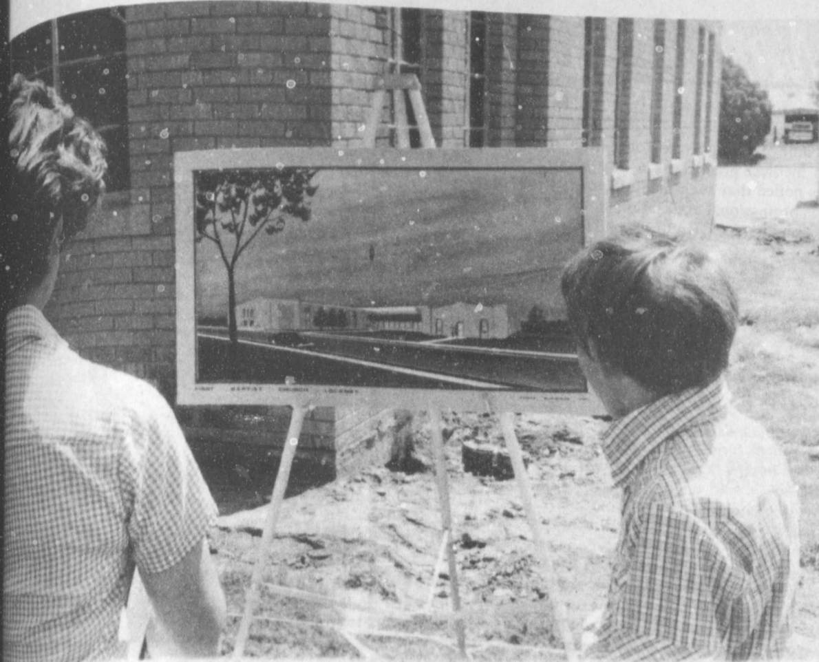
BREAKING CEREMONIES were held Sunday at the First Baptist Church in Lockney for a new educational building. The one story building, which will be attached to the existing sanctuary by a new covered courtyard, will take about four months to complete. Above church members look at an artists' drawing of the new building.
