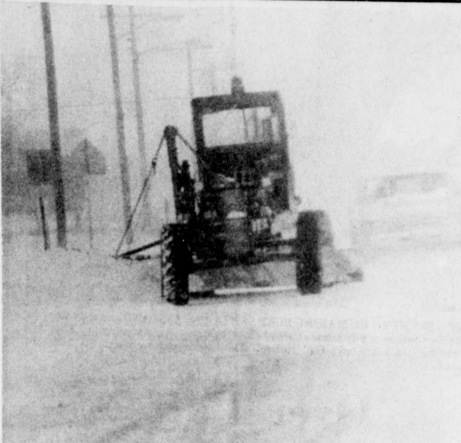
TEXAS HIGHWAY DEPARTMENT CREWS were out in force as Floyd County got another ten inches of snow for the second time in ten days. Winds gusting to 26 miles per hour reduced visibility to less than 50 feet at times.
