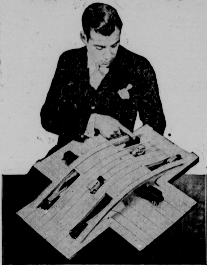
George K. Laham, twenty-four, of 37 Dent street, Boston, with the highway crossing construction model, which allows two-way continuous traffic at bad crossings. Note openings to permit autos to turn corners. Laham has studied the Hub traffic problem for the past three years.
