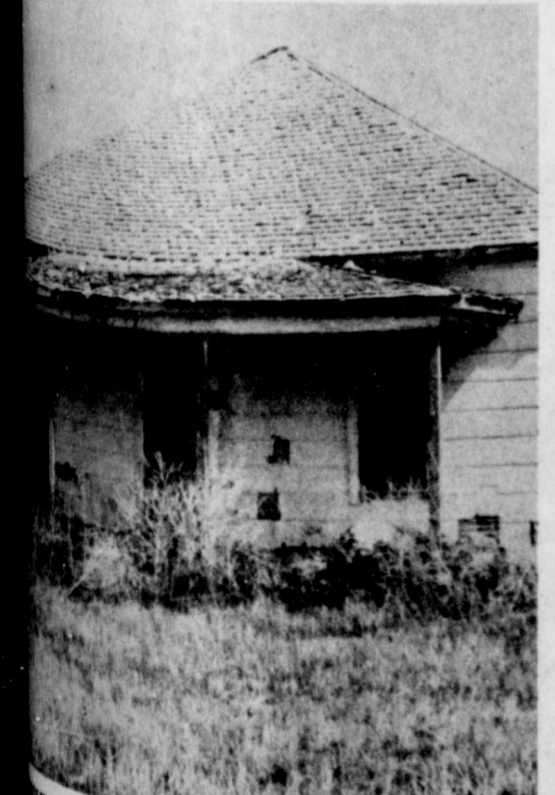
BEFORE DEMOLITION. This old house at Grover and 11th St., owned by the late Albert M. Jones, was torn out and the ground cleared helping to improve the appearance of the area.
