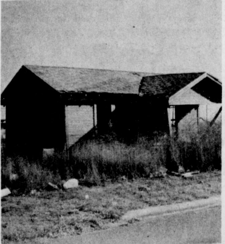
AFTER DEMOLITION. This cleanly scraped area with Della Plains school in the background shows how much certain sections of the city can be improved by taking out the old, rundown homes which are of no value.
