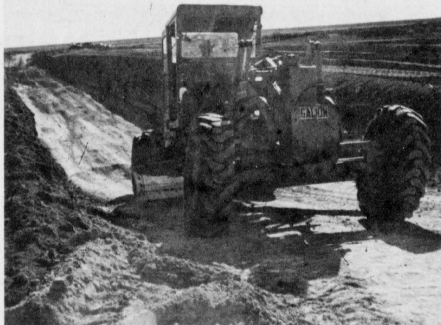
LONG HAUL — Ford Johnson brings his grader out of the new pit being dug by county workers at the dump grounds. This pit is about half completed.
