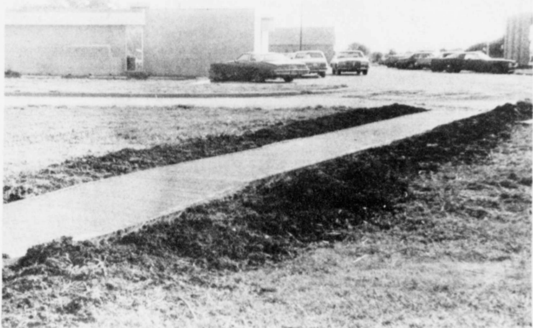
...fill it with good mix and sweep off the excess...
