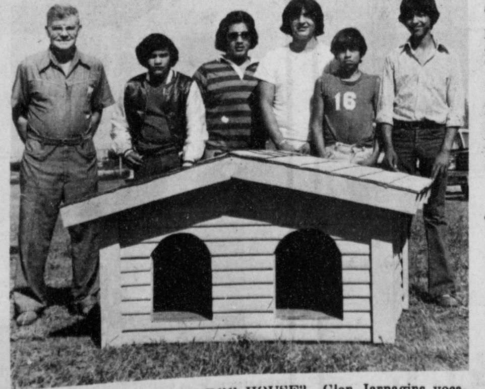
HOW ABOUT A DUPLEX DOG HOUSE?... Glen Jarnagins voca- tional general construction trades class has just finished this one for Joe Reid Jone's dogs...complete with hardwood floor. (l to r) Glen, Joe Reid Jone's dogs...complete with hardwood floor. (l to r) Glen, Felix Marmalejo, Joe Torres, Oscar Sanchez, Ricky Comacho, Albert (Staff Photo) Reio.
