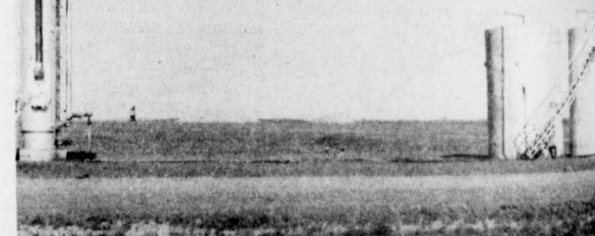
KENDRICK OIL WELL southeast of Lakeview is pumping mostly water. It is hoped that oil content will improve. Motor is powered by natural gas. Tank on left separates water and oil, storage tanks are pictured.
