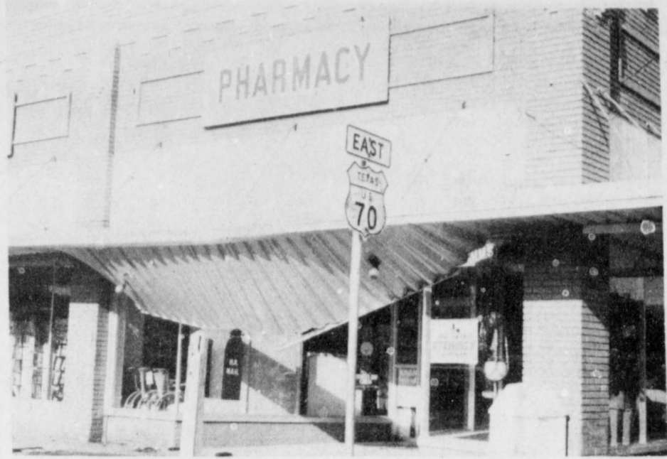
MONDAY NIGHT'S RAIN STORM demolished the overhead installation at Thompsons Pharmacy in downtown Floydada. This pharmacy located on Highway 70?hmmmmmm. (Staff Photo).
