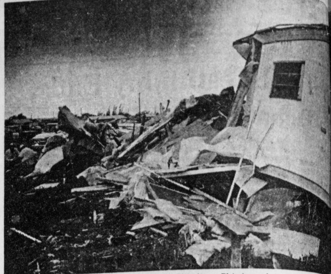
STORM DEBRIS—A tornado which raged through Plainview and struck the Lakeside Elementary School Tuesday left this trailer house in the 900-block of Joliet Ave. in ruins. Observers said the twister whirled about 50 feet from the ground through the Thunderbird addition of
