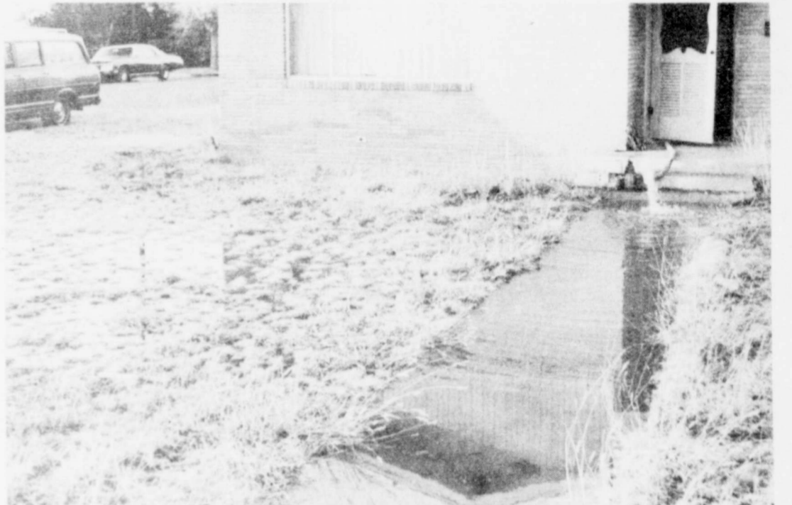
CLEANEST FLOORS IN FLOYDADA...but 31,000 gallons of water wasted. This brick home belonging to the late Robert F. Day sustained damages when water lines broke in the unoccupied home during the extremely cold temperatures in December.
