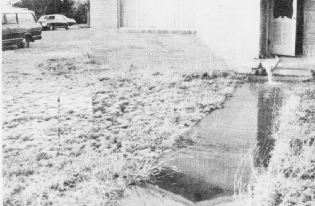
CLEANEST FLOORS IN FLOYDADA...but 31,000 gallons of water wasted. This brick home belonging to the late Robert F. Day sustained damages when water lines broke in the unoccupied home during the extremely cold temperatures in December. The water seepage was not discovered until last Saturday when a neighbor, Mrs. Alma Dunn, noticed her lawn was underwater. She called R. C. Day, a son, who lives in Floydada, however, he had no key to his father's house, so with the help of Sheriff Fred Cardinal, they broke into the house and located the problem. By that time 31,000 gallons of water had run through the meter since the billing in December. Mr. Day said there was 14 1/2 inches of water standing on the floors and it took four hours to pump 11 inches of that amount out of the house. They were still mopping up after the weekend. There was no estimate as to damage, but most of the flooring will have to be replaced relatives said. (Staff Photo)
