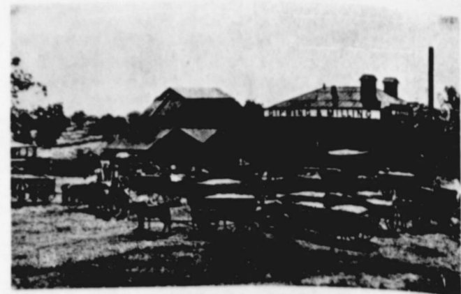
GINNING TEXAS-STYLE —By 1900, large gin operations began to become more commonplace. This one in Texas was equipped to turn out 100 to 200 bales a day, considerably reducing the time a farmer had to wait for his load of cotton to be ginned.
