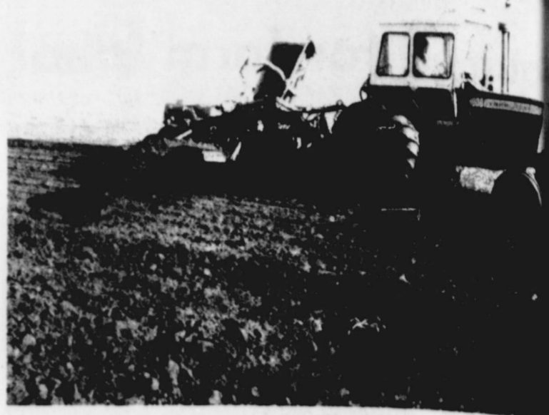
TERRACES UNDER CONSTRUCTION this week on the Lora and Henry Steid which is approximately 5 miles northwest of Morton. These terraces are shared under the Great Plains Conservation Program.
