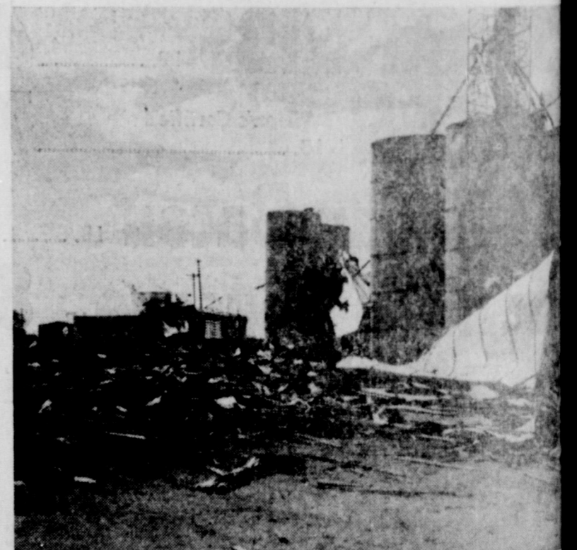
THE AWESOME POWER OF THE WIND wreaked heavy damage on grain elevator in Whiteface.
