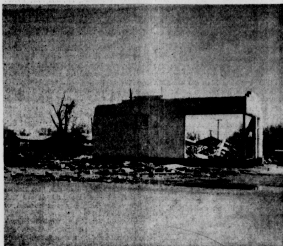
T. R. ROWLAND'S Gulf Station was a shambles following the blow. It is hard to believe that a parakeet and a mina bird in the building escaped uninjured.
