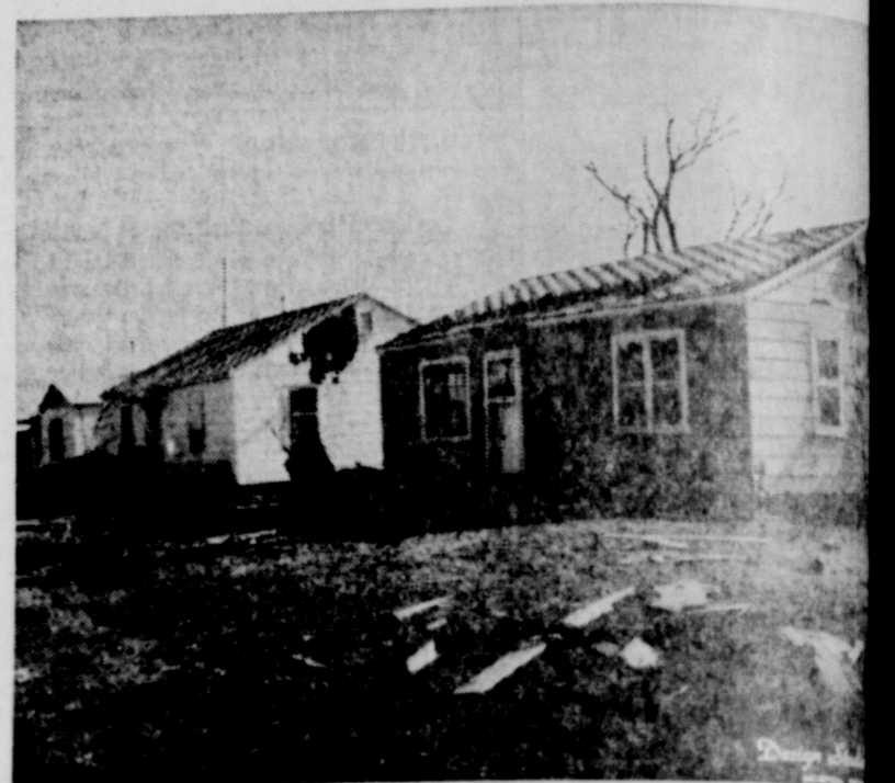
THIS ROW OF HOUSES adjacent to the school shows heavy damage by the force of the wind and flying debris.
