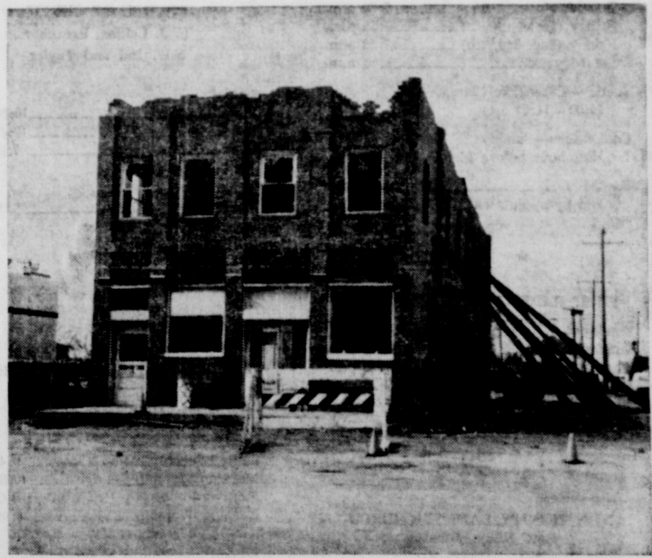
THE OLD WHITEFACE HOTEL building needed assistance in standing in the wake of the twister.
