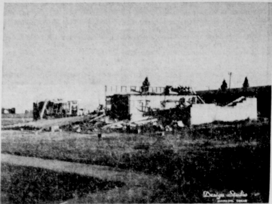
THE FORCE OF THE STORM smashed the Whiteface schools utility building to bits and pieces.
