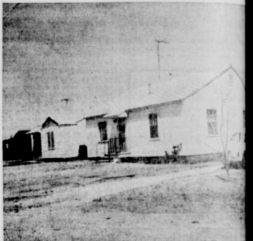
A MAJOR REPAIR PROJECT by their owners has caused these houses a fine appearance a year after they were struck by the storm.
