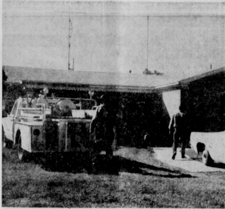
FARM HOUSE DAMAGED BY FIRE . . .
