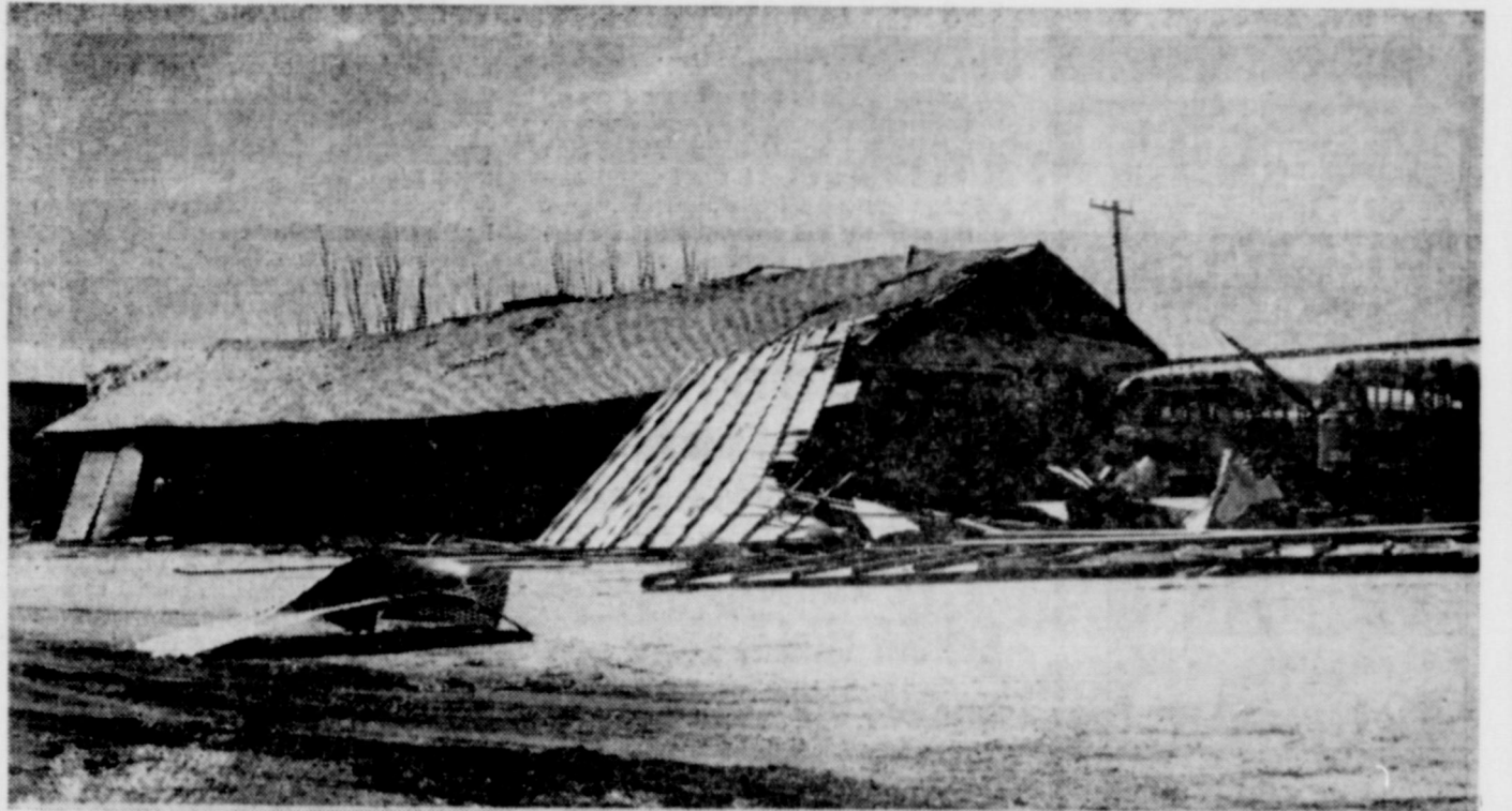
NORTH HALF OF BUS SHED carried away; south half collapsed on busses.
