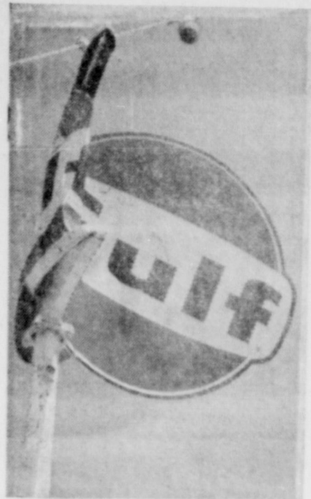
FORCE OF THE WIND wrapped this steel sign into a neat package.
