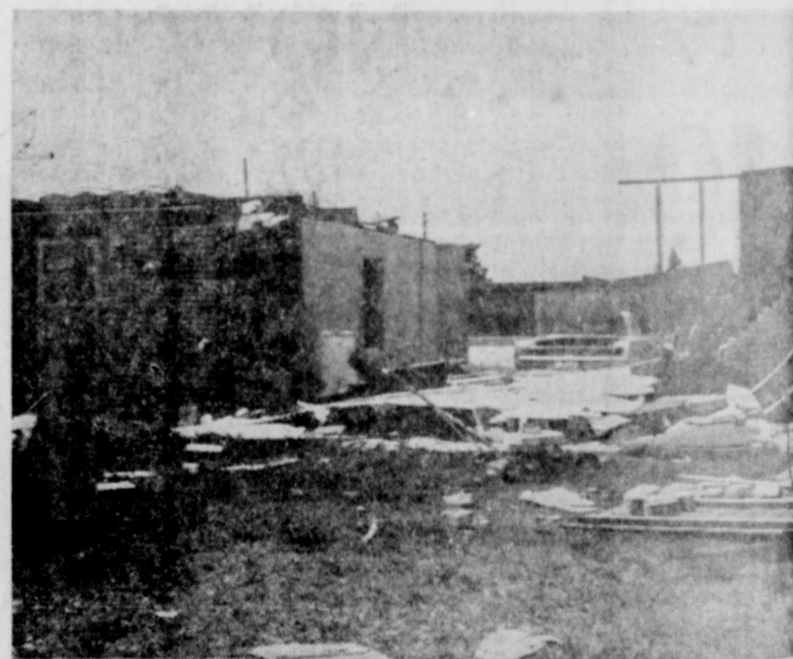
THE ALL-BRICK HOME of the Olin Lewises is a total loss.
