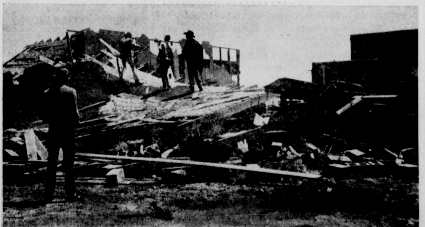
THE WHITEFACE SCHOOLS utility building was smashed to bits and pieces.
