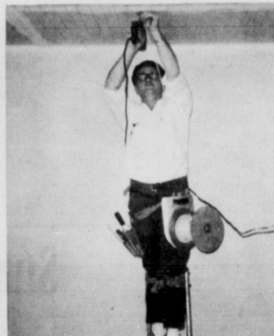
Doug Kelley, right, is shown as he installed the electric ceiling cable to provide electric heating for Dr. and Mrs. Roden's new home.
