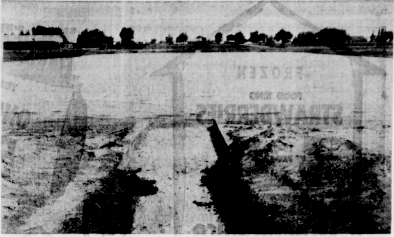
THE RECENT RAINS around Morton have succeeded in filling Strickland Lake to the brim. The photo, made Monday afternoon, shows the new concrete spillway that was installed recently to prevent erosion when water drains in to the lake. (Staff photo)
