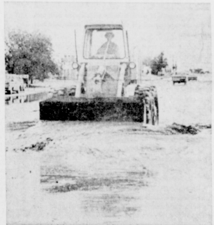
Mud being removed from N. Main in Morton
