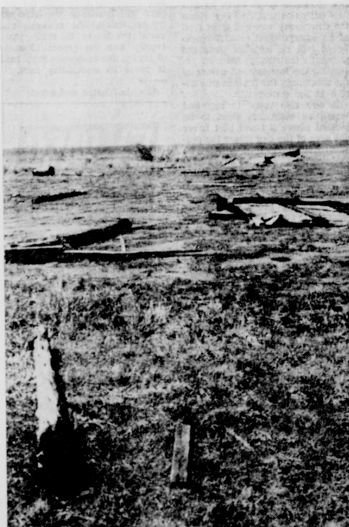
Fence post uprooted
