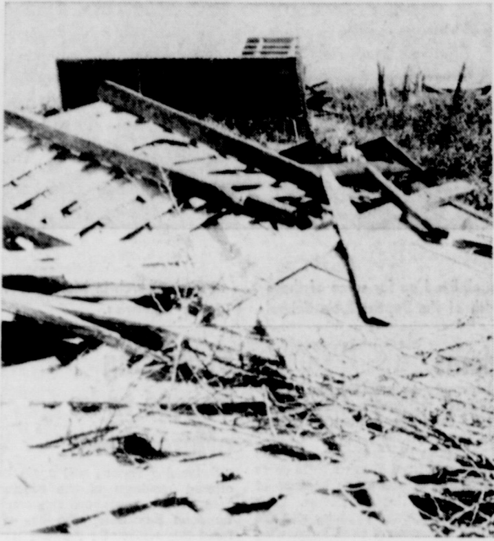
Some repairs needed
