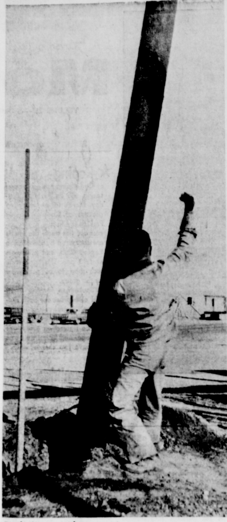
Replacing a pole . . .
