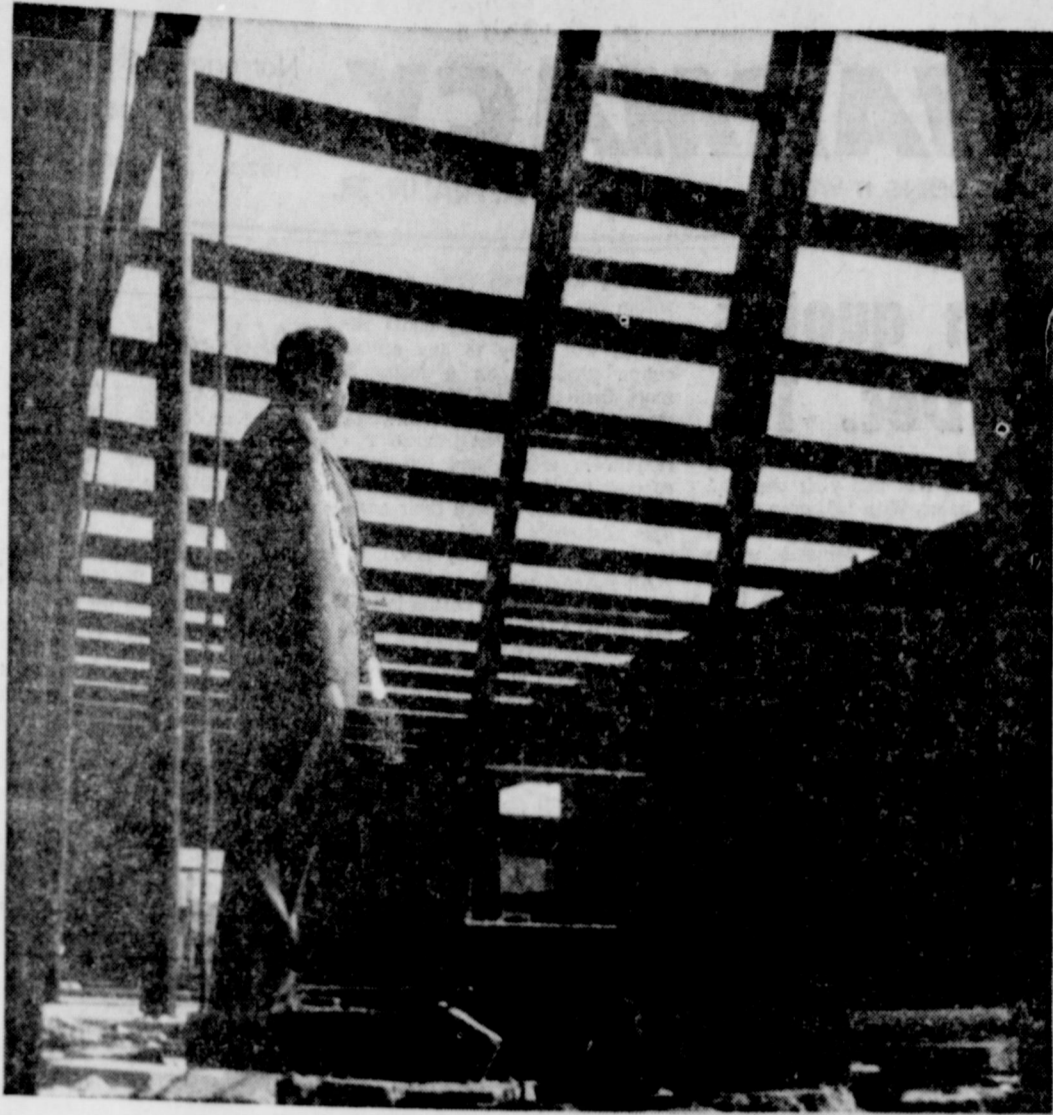
Building nears completion
