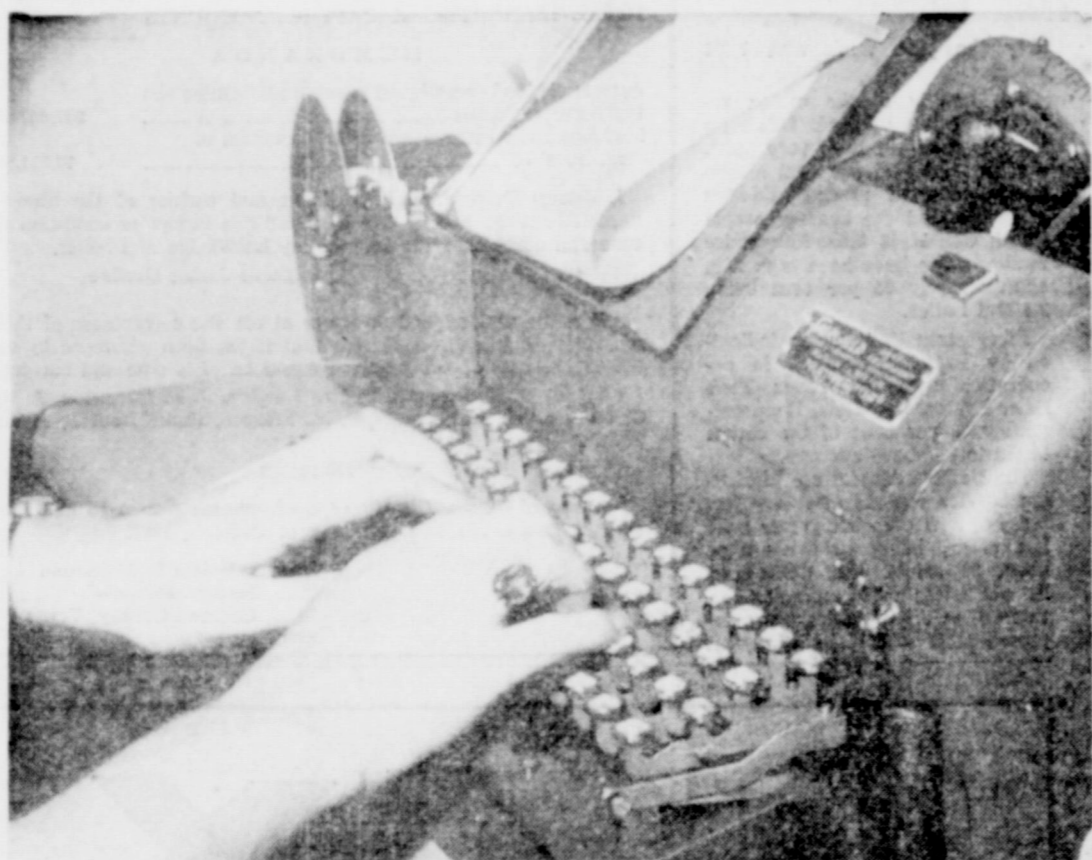
Tape is punched to cast the type
