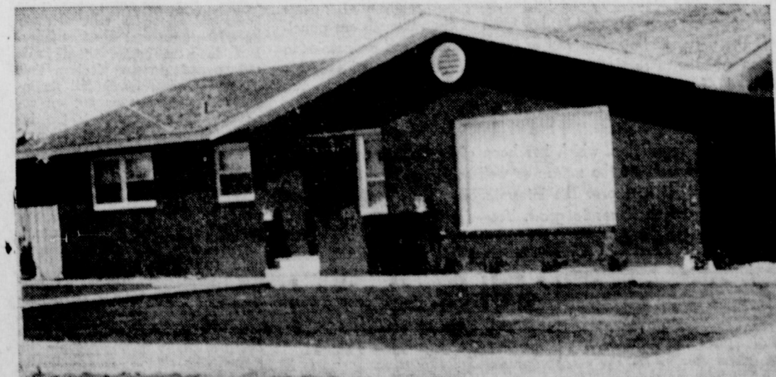
MR. AND MRS. A. R. McDANIEL built this red brick on South Main. It with two others
