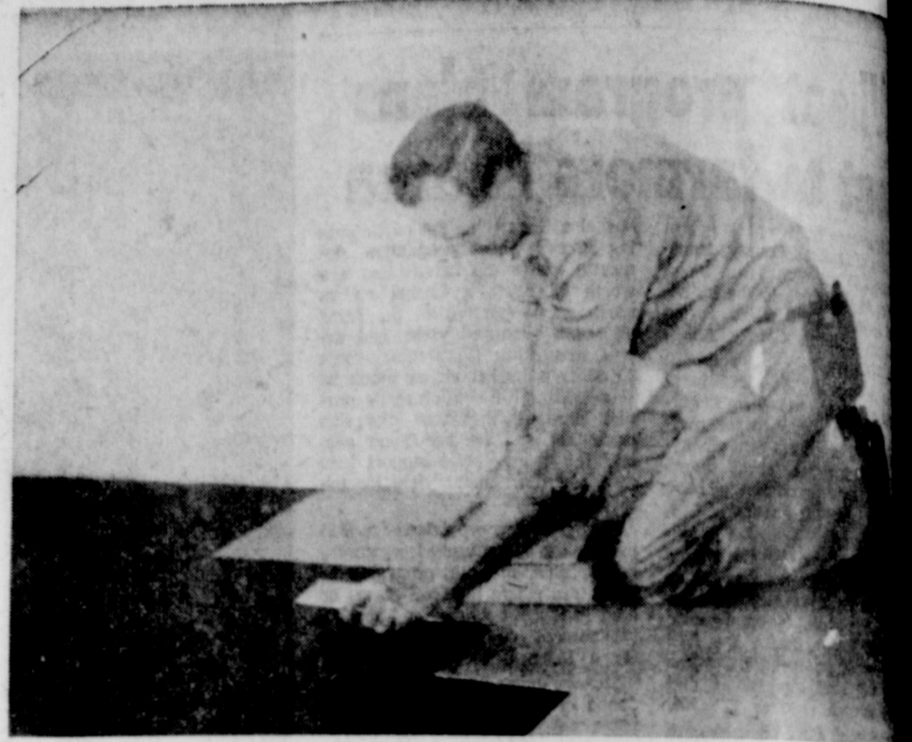
Floor installation in new high school
