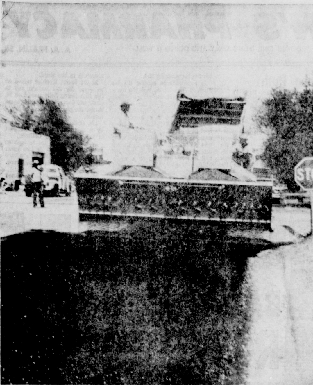
Paving work in progress
