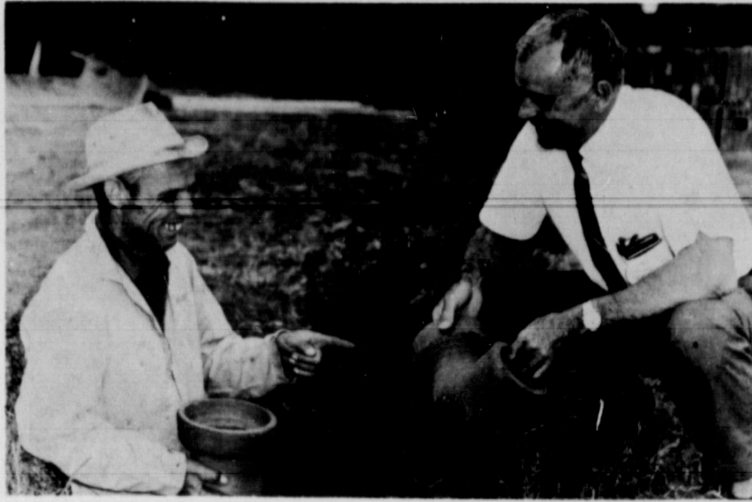
MILESTONE REACHED . . . Pete Hollis, superintendent of Friona's sewer department, points to the sewer tap which made number 1,000 since the city's sewer plant was put into operation in 1950. City Manager A. L. (Jake) Outland looks on.
