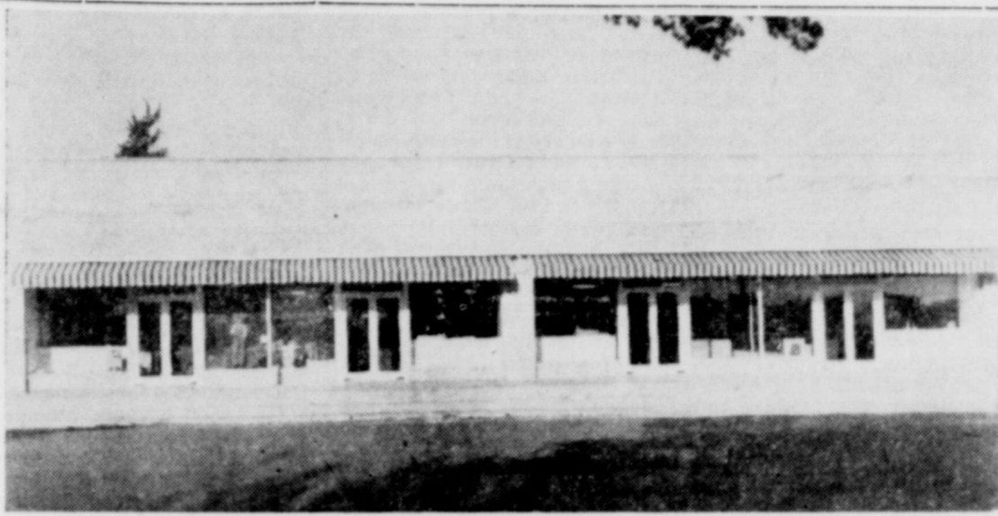
Remodeling has been completed on St. Clair's Department Store, pictured above. The building is 84x128 feet and covers 10,752 square feet of floor space.
