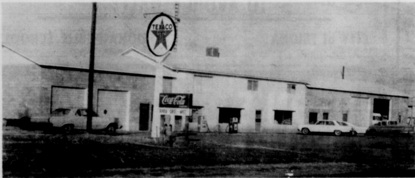
Newly Remodeled Facilities At Rhea Store.
