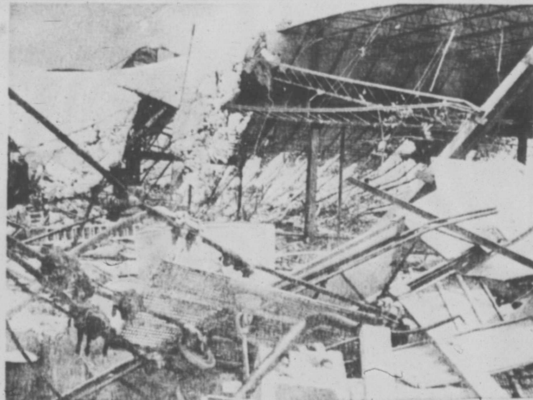
ALL THAT'S LEFT--This was a grocery store in a shopping center at Gulfport, Miss., until Hurricane Camille struck Aug 17. This photo was made by Beacon-News Editor Dalton Wood last Thursday (See Woodwork column at left).
