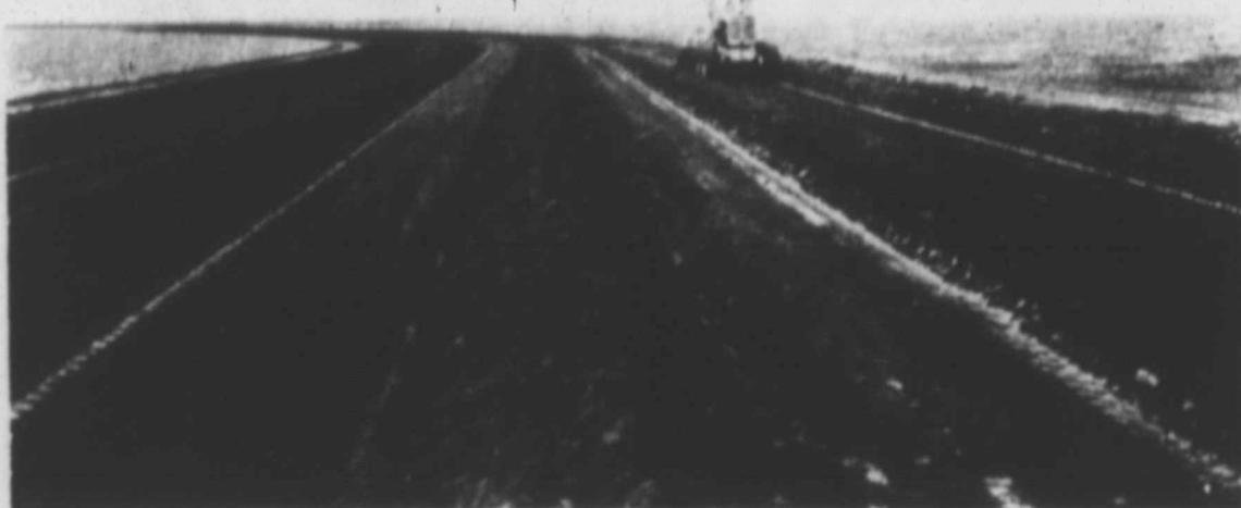
Farm near Springlake in the process of being bench leveled. The benches are being constructed on land that has about one and one-half to two feet fall per 100 feet.
