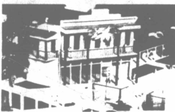
Old Building Restored on Site
