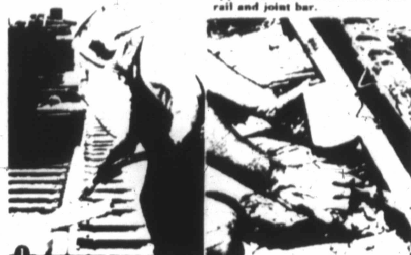
1 (Above) Joint bars and rail ends are sandblasted prior to application of epoxy glue.
