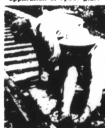
3 (Above) Joint bars are replaced and bolts tightened.
