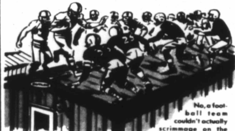
No. 6 football team couldn't actually scrimmage on the roof. But the building—produced by Butler Manufacturing Co.—is strong enough to take the weight of an entire team and more, if evenly distributed.
