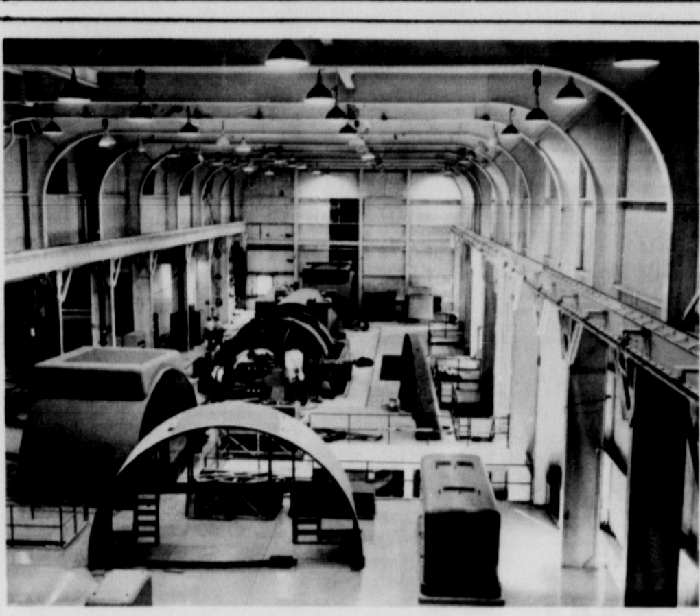
Pictured under construction at Southwestern Public Service Company's Plant X, in Lamb County, is a 210,000 kilowatt generator. The largest unit ever installed on the company's system, the huge turbo-generator will go into service in mid-1964. Southwestern Public Service Company has announced that 1964 will be a record year for investment in construction and new facilities, with $30,222,000 budgeted for improvements.
